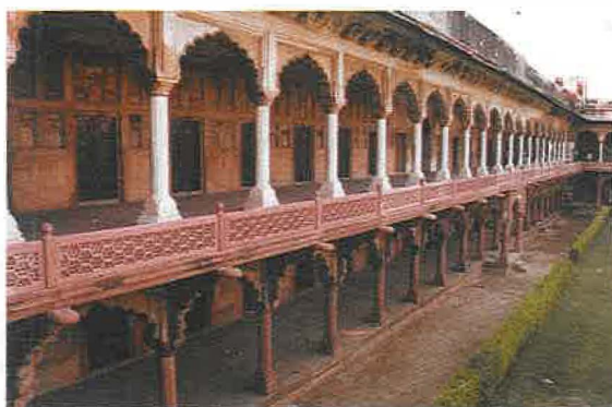
Machchhi Bhawan, Agra Fort after fixing red sand stone jali railing.
